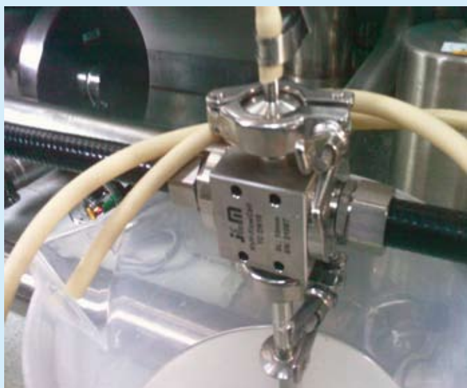
Fig.1: Online installation for cleaning validation in a pharmaceutical process
